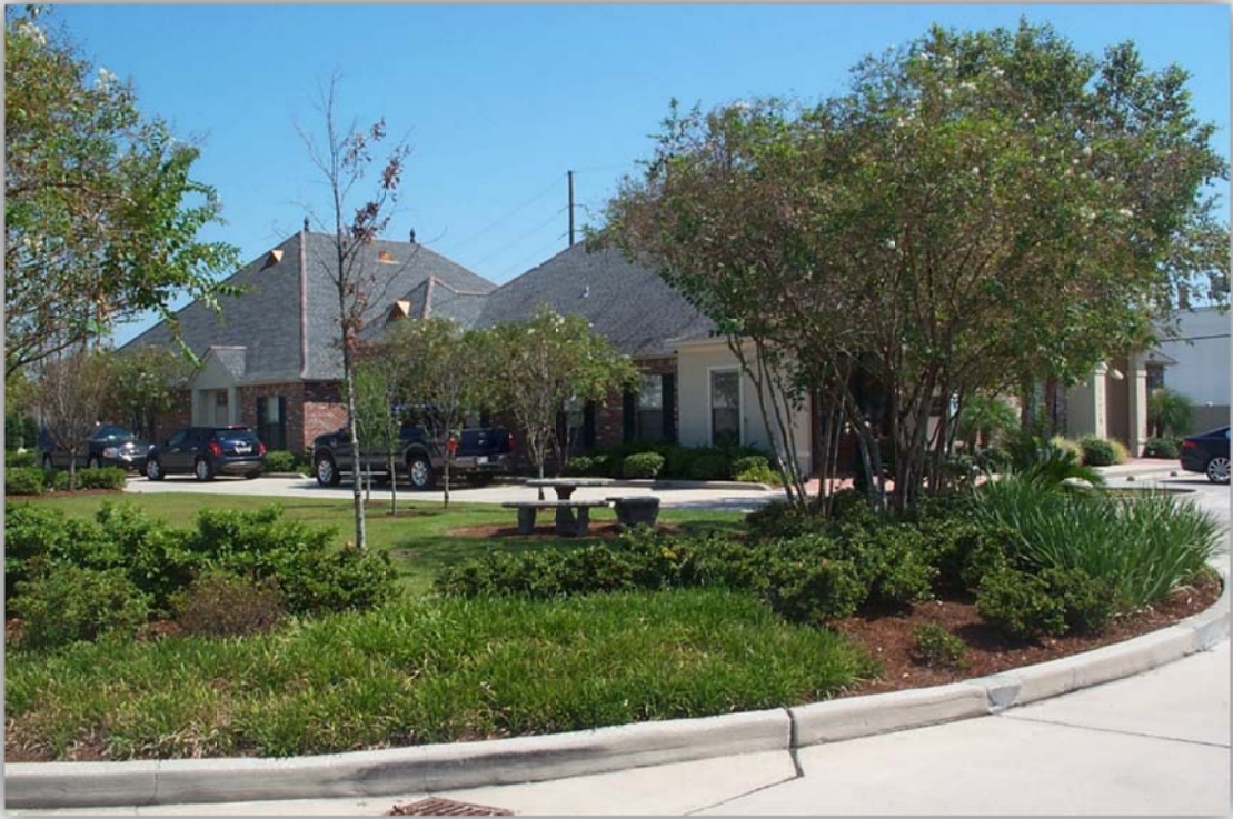
Office Park Grounds
